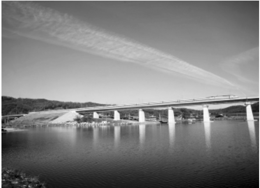
KTX train running on bridge
